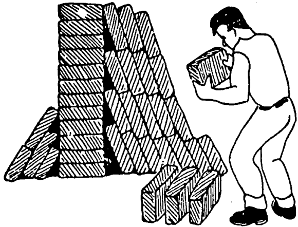
Figure 46. Adobe block is stacked after a month of curing.
