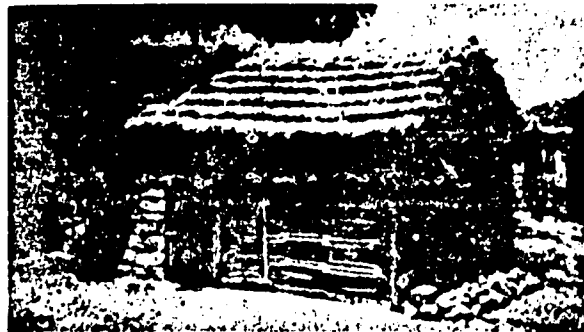
Figure 4. The right half of this residence in Greece shows the wattle in place. Daub will follow.
