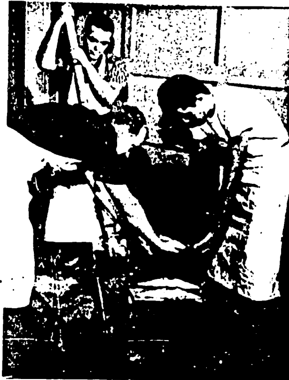
Figure 54. Charging mold box with soil mix.
